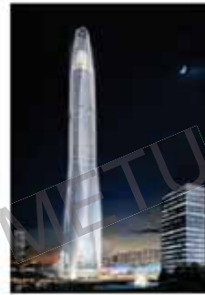
11 CTBUH, among completed, stacked and architectural topologies. 12 Next Generation Supertall Tower Form Determinants: A study of the Tianjin CTF Finance Centre, 2016, CTBUH
